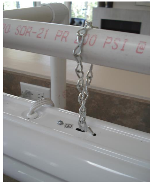
Figure 3 Detail of chain and "S" hook attachment
